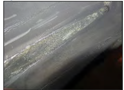
Fig. 4. Bacteria in cracks in liner
