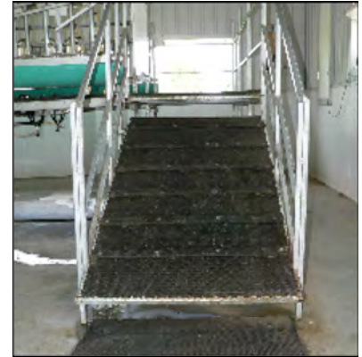
Fig. 8 Ramp to parlour is well-lit and secure
