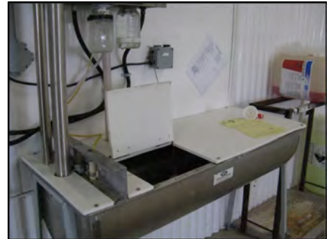
Fig. 52 Covered wash sink helps maintain temperature of wash water
